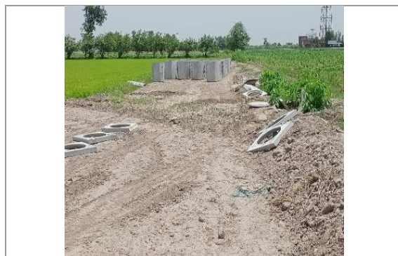
Figure 4.56: Improper placement of Segments & Naccas on watercourse no 21600-R
