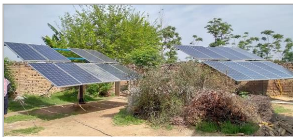
Figure 4.40: Solar System for Tube well of Shah Hussain Mera Badhaber, District Peshawar
