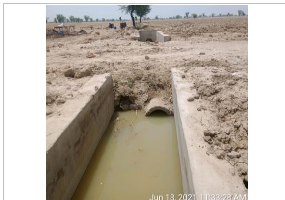
Figure 4.91: Concrete Culvert with Watercourse
